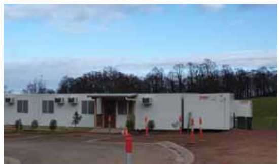
The temporary building on a paddock in Kinglake where Colleen has worked with other psychologists, social workers, GP s and community workers.
